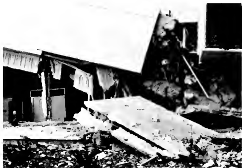
Photo 27. Precast concrete wall panel on ground fell from supporting structure at emergency entrance (basement level).
